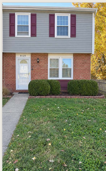
● AFTER: ON THE SITE
